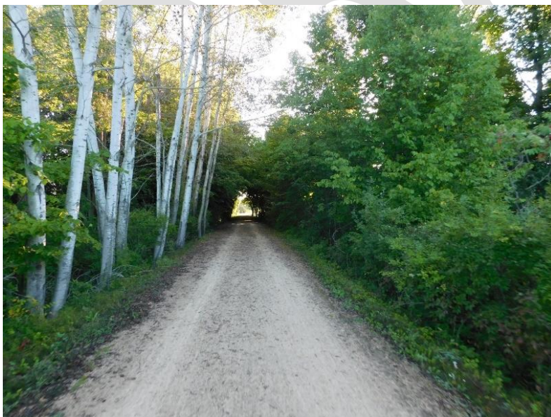
Figure 8. Option B2 would require moderate vegetative removal and grading to construct Trail Type 2 (Separated Snowmobile and Cross-Country Ski Trails).
